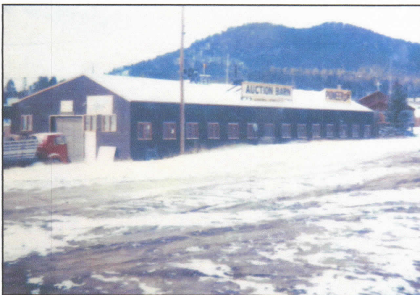
After its life as the granite works, the building was An auction house. This photo gives an idea of the dimensions of the building, along with all of its windows.
